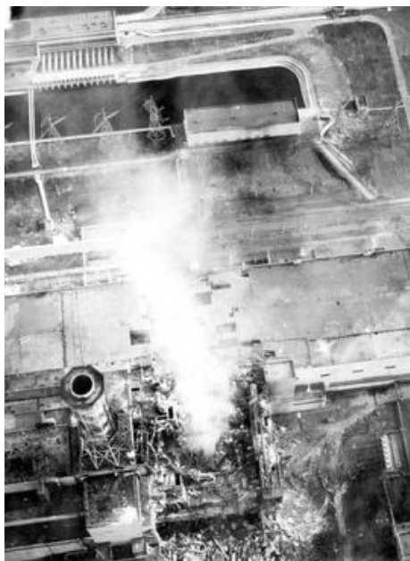
Figure 18. Smoke from Chernobyl number 4 reactor burning. Aerial view. Photo Credit: Wikipedia.
