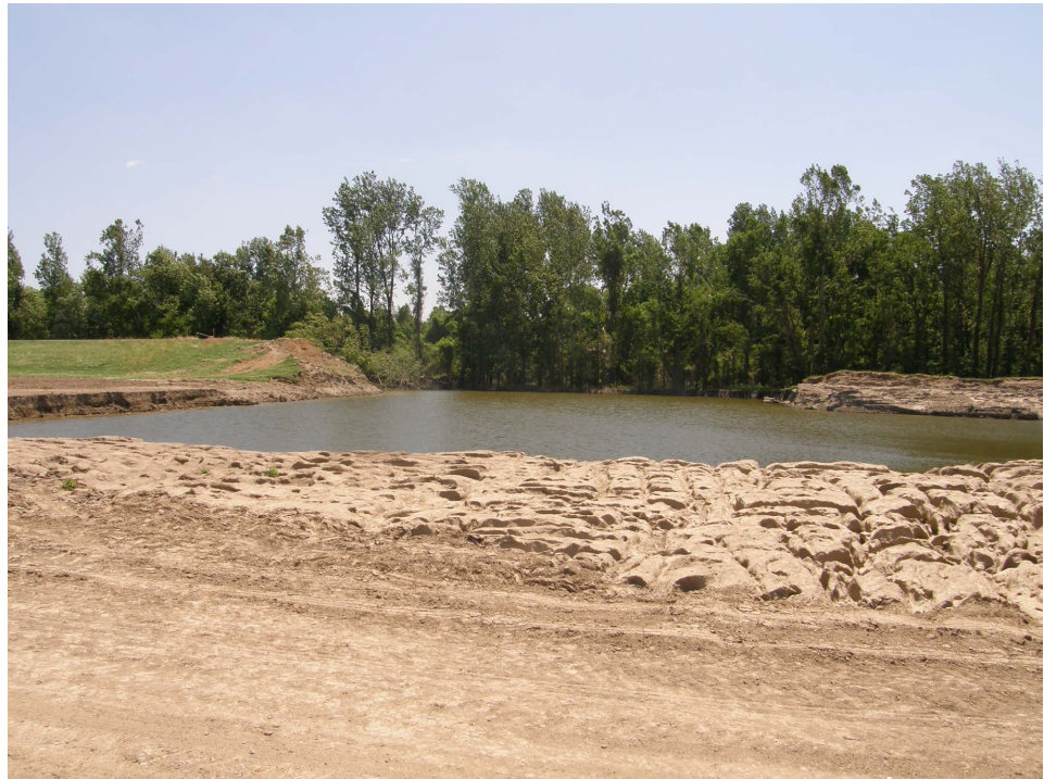
Figure 8. The Birds Point levee breach created a crater lake that extended many meters through the levee.
