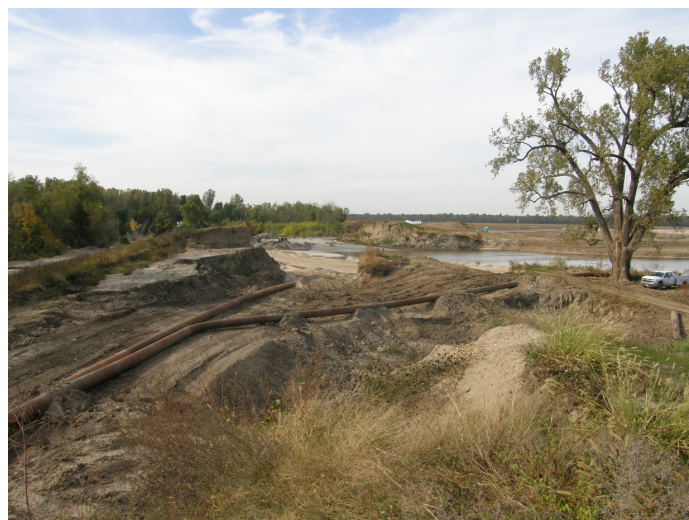
Figure 11. A crater lake was formed at the Big Oak Tree frontline levee when the fuse plug was blown and floodwaters rushed into the floodway.
