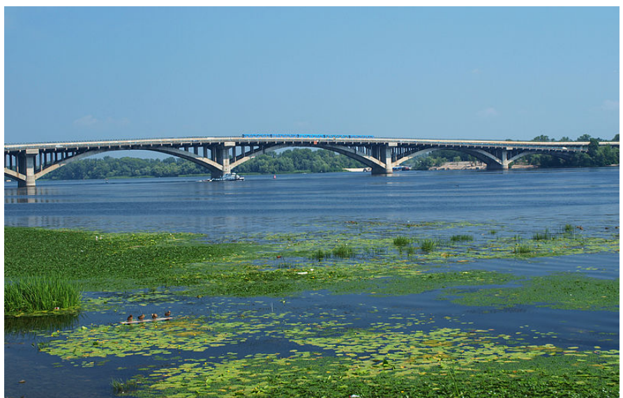
Figure 22. Bridge over the Dnieper River in Kiev, Ukraine. Photo Credit: Petar Milosevic.
