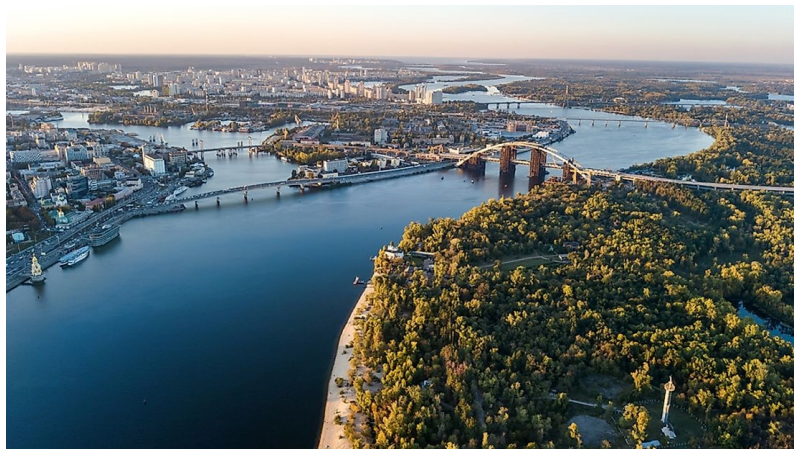
Figure 4. Four motor bridges and one railroad bridge over the Dnieper River in Kiev, Ukraine. Photo Credit: Encyclopedia Britannica, Cavan iStock/Getty images.
