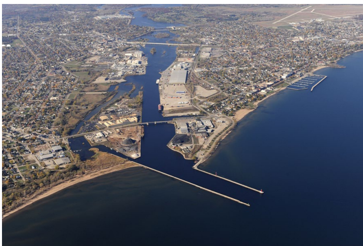
Figure 14. Aerial view of the former Ansul company chemical plant on Menominee River in Marinette, Wisconsin (L) and Menominee, Michigan (R). The Menominee River flows into Green Bay. Published with copyright permission from Editor of Open Journal of Soil Science.
