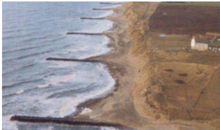
Figure 11. Groyne battery: long term solution [4].
