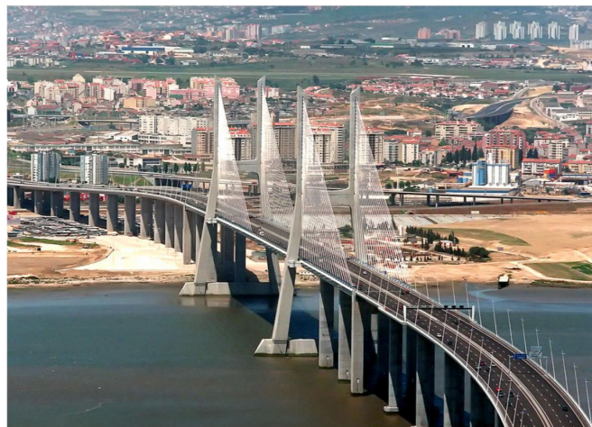
Figure 6. General view taken from central viaduct towards main cable stay bridge [3].
