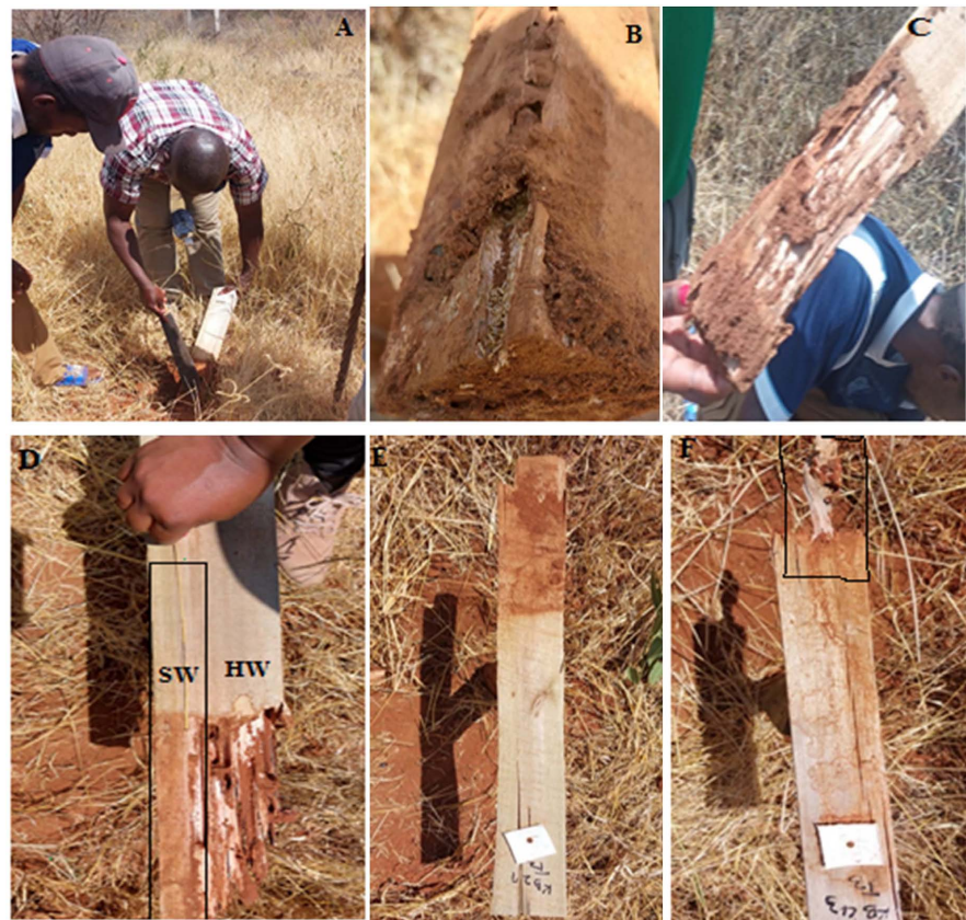
Figure 4. Illustration of observed damage caused by termites and fungi. 20 kg/cm 3 water based chromated copper arsenate (CCA) treated sample assessment (A), termite activity on heartwood of a 20 kg/cm 3 CCA treated sample (B), 20 kg/m 3 CCA treated sample with a combination of fungal and termite activity (C), an attacked heartwood (HW) and an intact sapwood (SW) (D), an intact 6 kg/m 3 CCA treated sample (E), a control group sample showing higher damage level.
