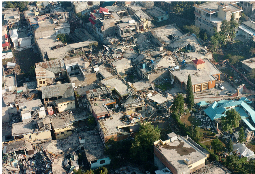
Figure 6. Photograph of the town of Muzaffarabad, near the quake epicenter. Muzaffarabad recorded the highest human loss in a single day and the most extensive damages in its history. The whole city needed to be rebuilt [24].
