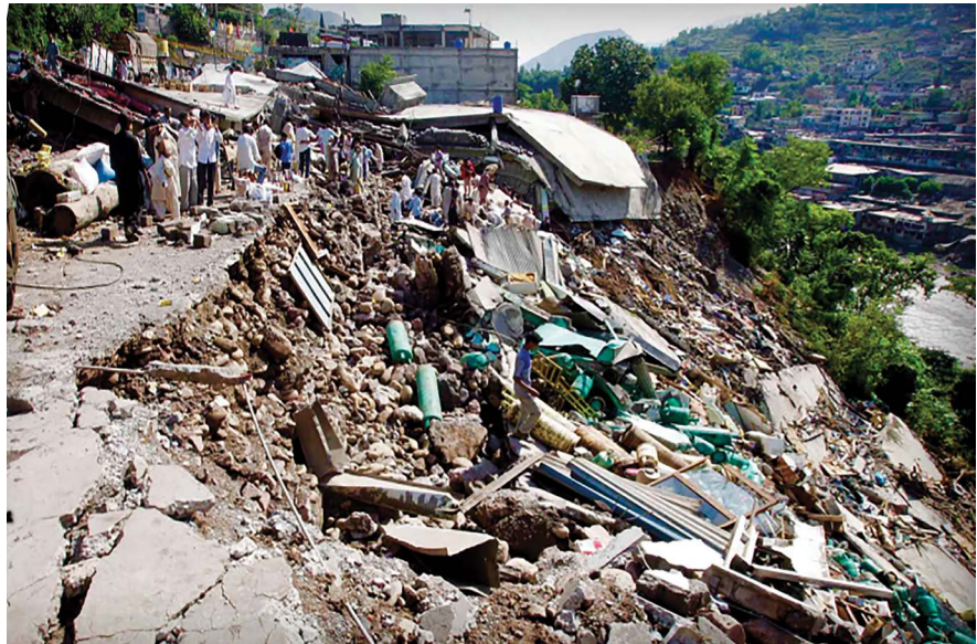
Figure 2. Destruction of structures and hillslopes in Muzaffarabad, near the earthquake epicenter. It was the most devastating earthquake in the history of Pakistan since its birth in 1947 [15].
