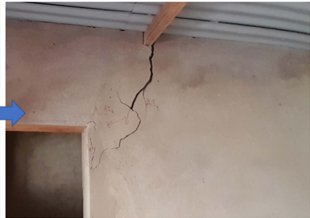
Photo 2: Adobe. Transformation of intermediate cracks into structural crack. June 2023 Richard Z. June 2023
