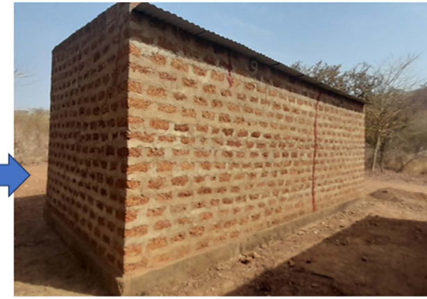
Photo 10: Exterior view of the cut laterite bricks' witness habitat in June 2023. Richard Z. June 2023
