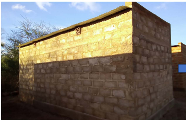
Photo 7: Exterior view of the breeze-block witness habitat in June 2022. Richard Z. June 2023
