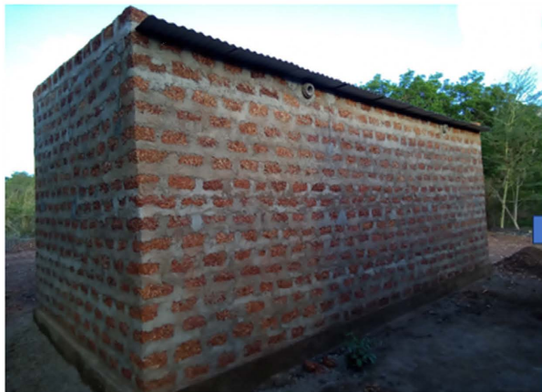
Photo 9: Exterior view of the cut laterite bricks' witness habitat in June 2022. Richard Z. June 2022
