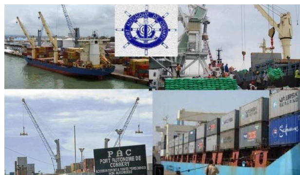
Figure 1. Some parts of the autonomous port of Conakry.
