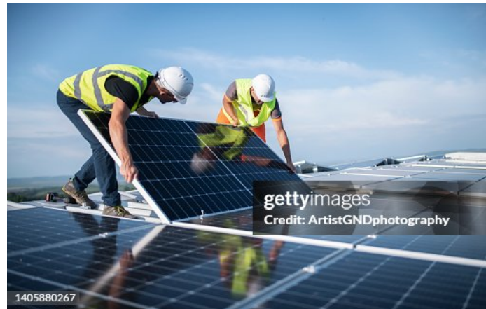
Figure 12. Below displays solar plant installation (Source: Solar power station, Getty images).
