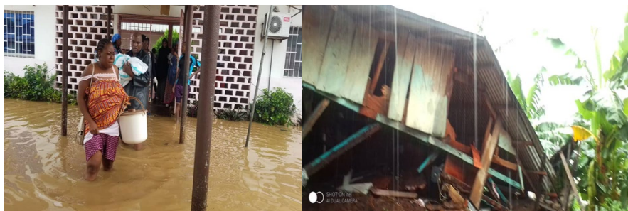
Figure 1. Showing flooding in Limbe (Source: Author's original picture).
