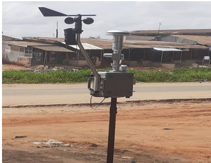
Figure 2. Air monitoring at the impacted neighbourhood Lapeleko on the 26th of March 2024 with ARA N-FRM.
