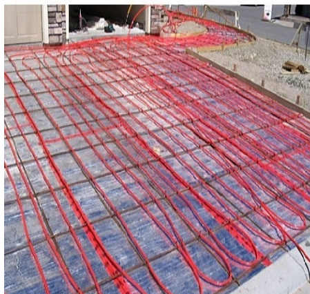
Figure 6. Installation of hot water pipelines in parkway for snow melting.
