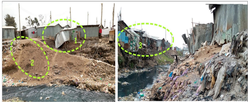
Figure 1. House location in vulnerable setting (Source: CGN, 2023).
