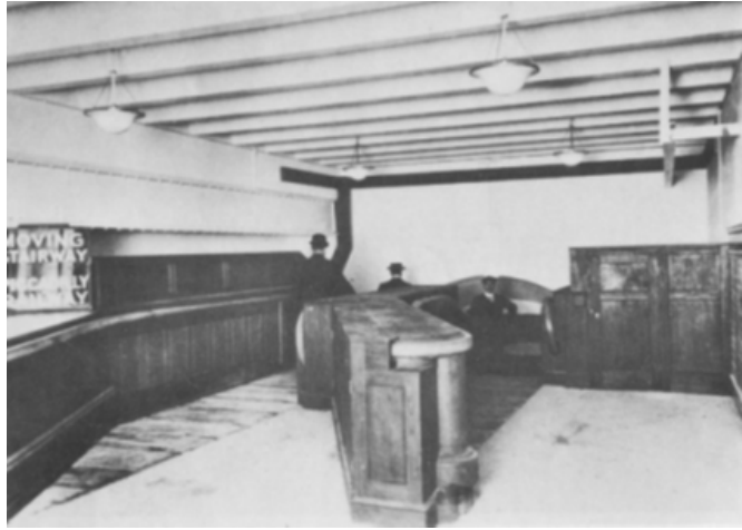
Figure 16. “Seeberger” flat-step escalator and note barrier deflector (reproduced from Elevator World Magazine , January 1992) (Strakosch & Caporale, 2010).
