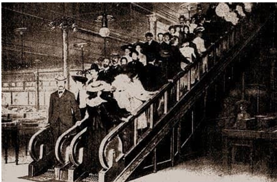
Figure 10. Early type of the Reno's escalator (Fenzel, 2021).
