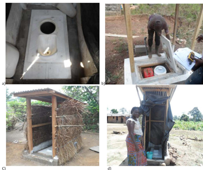
Figure 2. Photographic illustrations of excreta collection equipment: a) stand and bowl in Salifoukro, b) interior of pit in Simmimbo, c) completed latrine in Blanfla and d) completed latrine in Kouakoublékro.
