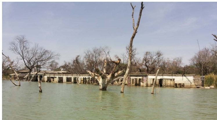
Figure 2. Flooding out of business premises.
